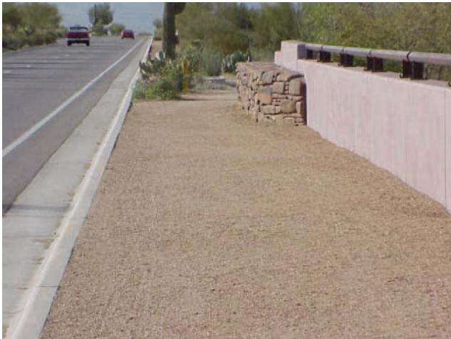
Bridge Over Main Wash
