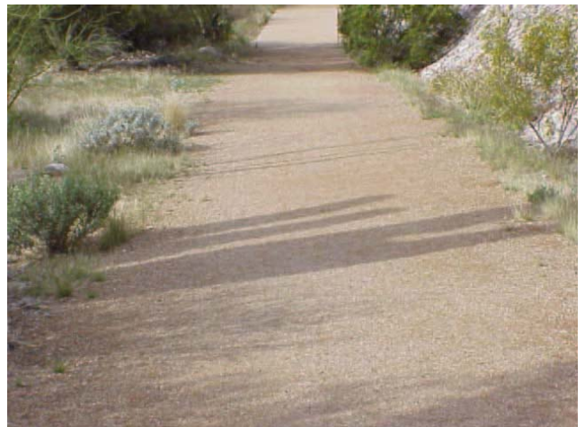
Stabilized Decomposed Granite Trail
