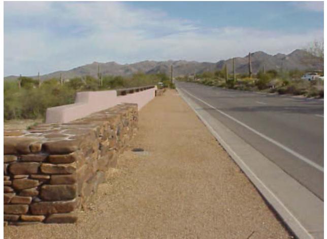
Bridge Over Main Wash
