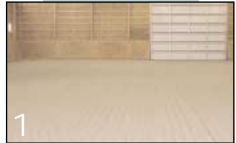
Base material before application
