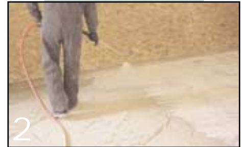
First application of Soil-Sement* Engineered Formula (SSEF)
