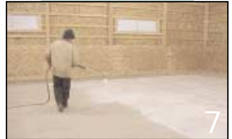
First top seal coat of Soil-Sement® Engineered Formula
