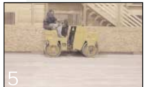
Compaction of base with Soil-Sement* Engineered Formula
