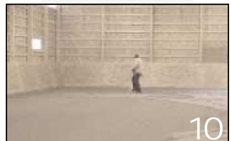
Treatment of footing with Arena Rx®
