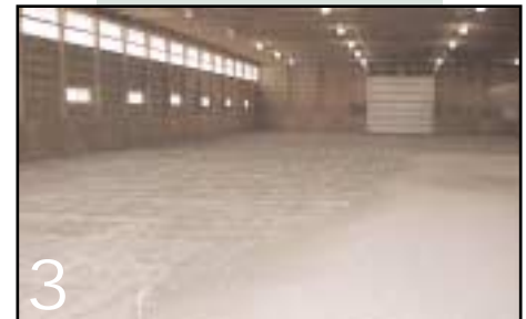
Left side is the treated base, right side is the untreated base
