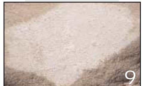
Cured Base-Bldr™ underneath the footing
